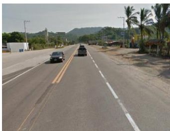
Carretera Federal No. 200 Tepic – Puerto Vallarta.
