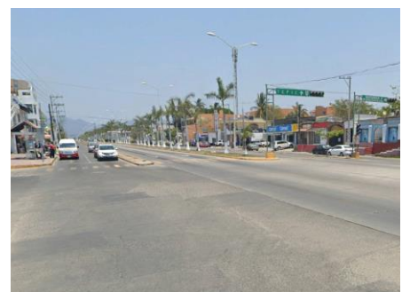
Carretera Federal No. 200 Tepic-Puerto Vallarta
