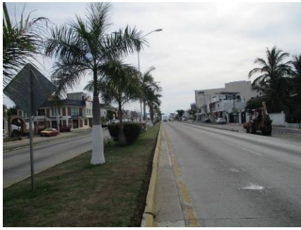
Carretera Federal No. 200 Tepic - Puerto Vallarta
